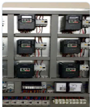
Inside the panel
