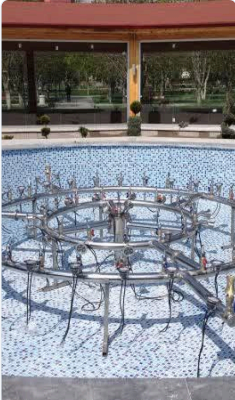
Ring manifold installation
